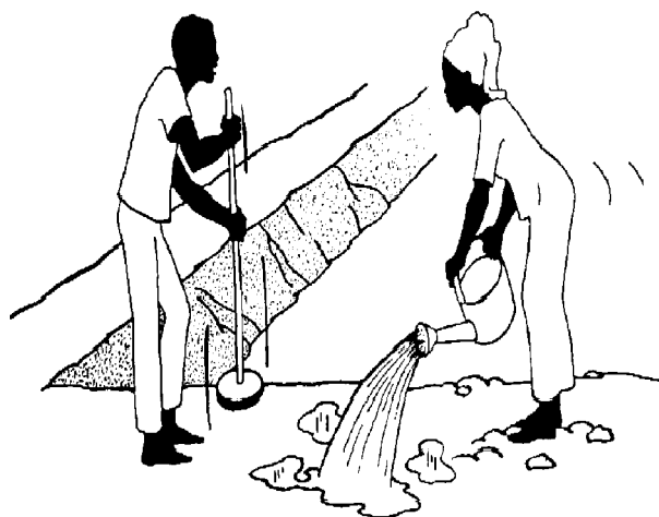
Figure 13: Compacting the dike (Viveen et al., 1985)
