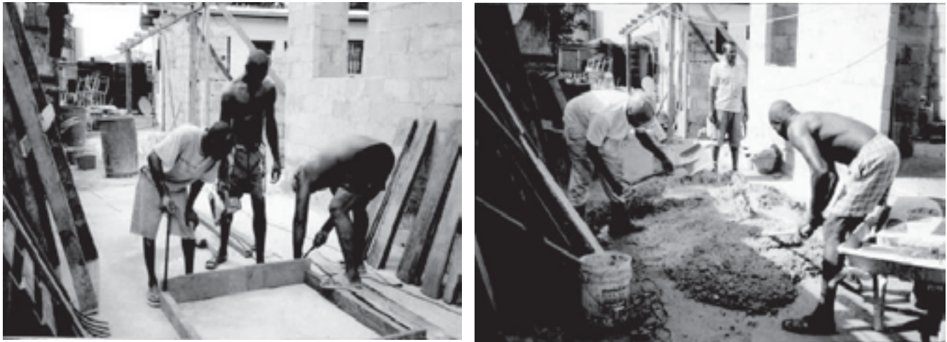
Pastor Awong and some ex-inmates at work on the construction site
