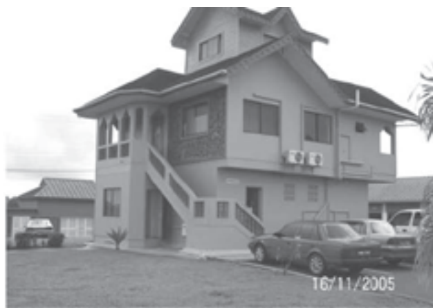
One example of a renovated office building at the PEC compound
