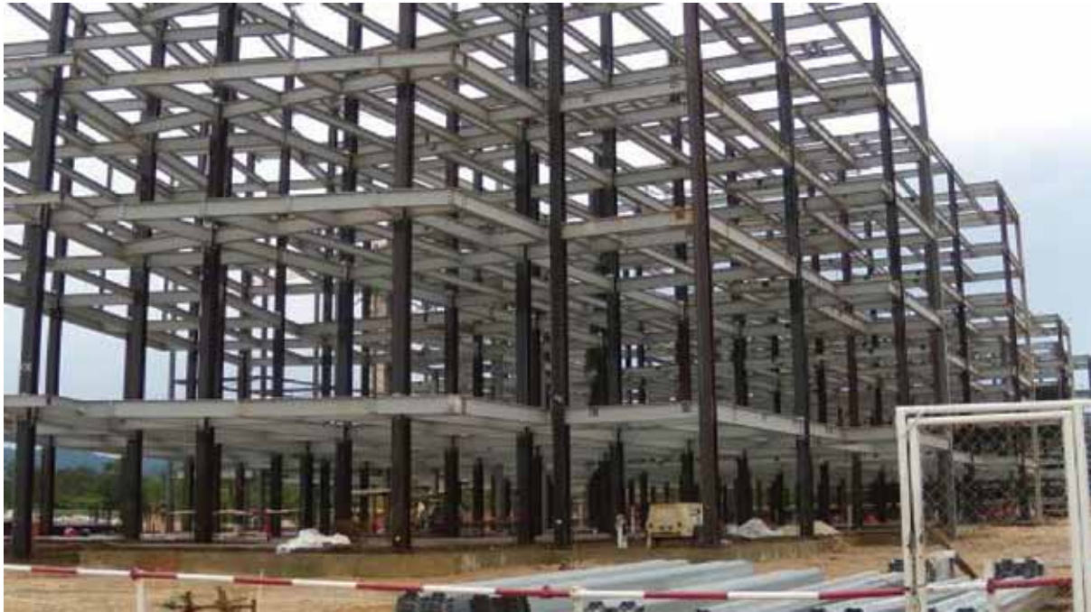
Signature Building Complex under construction, September 2009.
